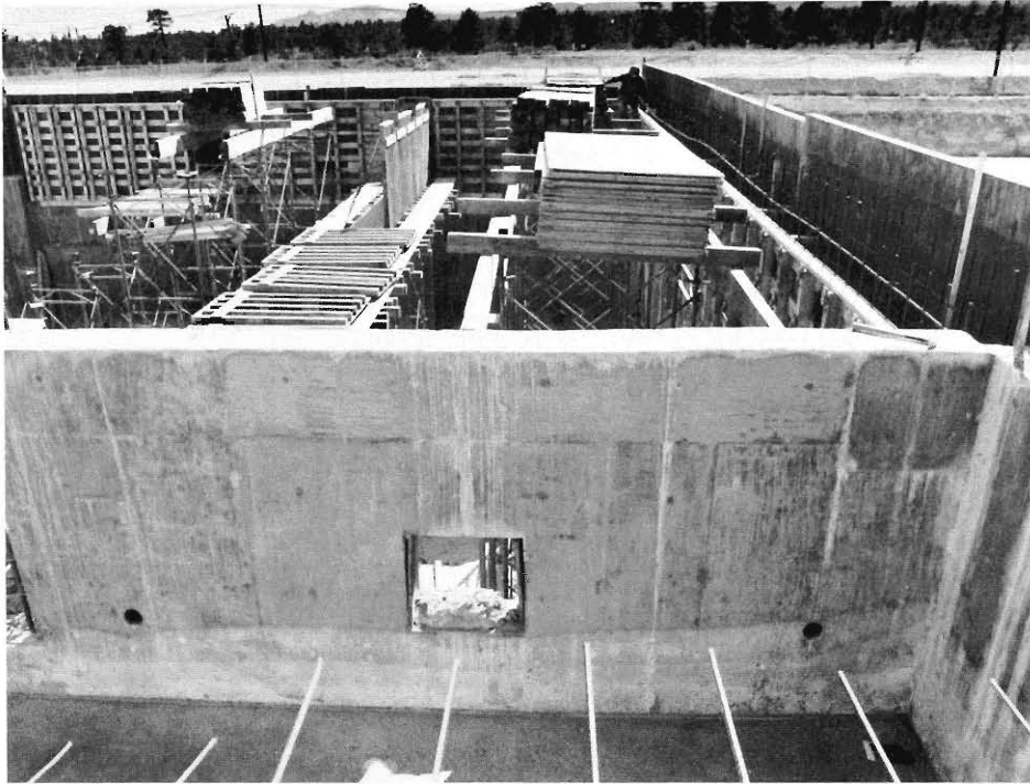
Harold helped convince the AEC of the absolute necessity for a new plutonium research and development facility. Construction started in 1974.
